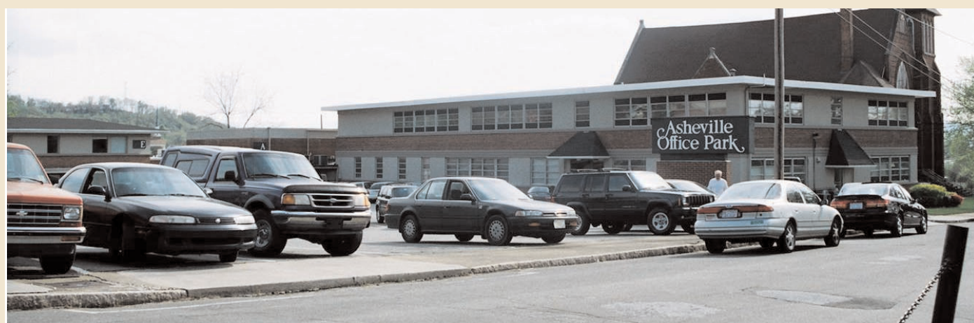
Allen High School, now Asheville Office Park, was founded by the United Methodist Church in 1877 and for almost 100 years served as a premiere education facility for African American Women. Having closed its doors in 1973, it is now the Asheville Office Park on College Street. Center for Diversity Education Archives
