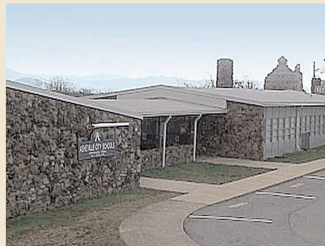
Lucy Herring School is now the Central Offices for Asheville City Schools
